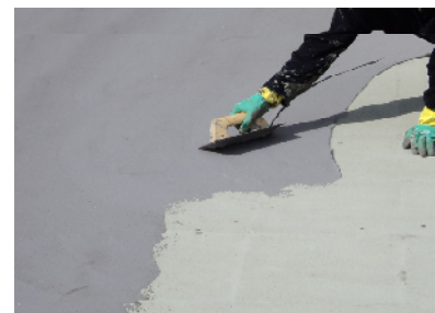
...with a flat trowel on horizontal surfaces.
