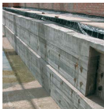
Concrete repair in the most difficult of conditions.
