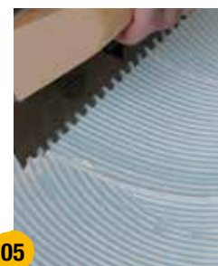
05 Lay the ceramic or mosaic tiles using ELASTICER .
