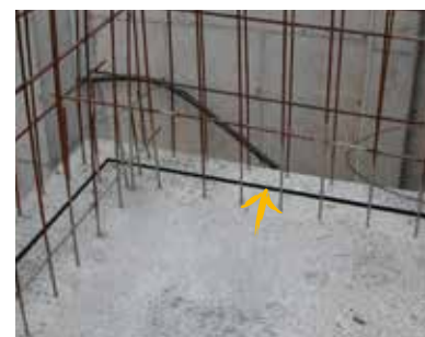
Application of FUGA-STOP 25 x 20 mm
