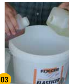
03 Mix the 2 liquids of the 3-component ELASTICER .
