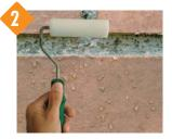
Apply 2 coats of FIX-WALL using a varnish roller (let dry for 24 hours between coats).
