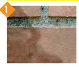
Without protection, facing brick absorbs rainwater, which will end up seeping inside.
