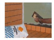
For floors in general, you can also use **EUROCOLOR FLEX** for grouting. However, for floors that make up ceramic shower trays you should always use **CERPOXI.** Its main characteristic is that it is 100% waterproof and antiacid. They are pre-dosed epoxy resins that are very liquid and are formulated to be applied manually with a rubber trowel such as **FIX-LLANA** or with a rotary machine in industrial installations with a great number of square metres.
