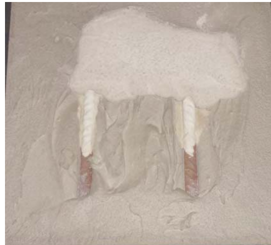
When FIX-REPAR ANTI-OXID turns to a light gray color, we can apply the repair mortar FIX-REPAR R2 or R4 .
