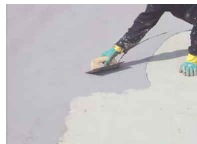
...with a flat trowel on horizontal surfaces.
