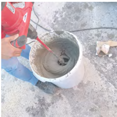
According to the projecting machine that we use, we will have to mix it previously with just water.
