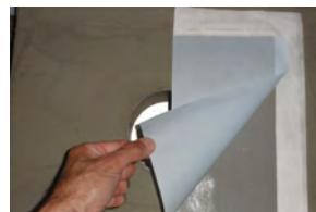
Fold the sheet on the other side of the pre-cut.
