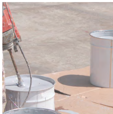
Mix with an electric mixer for 2 minutes.
