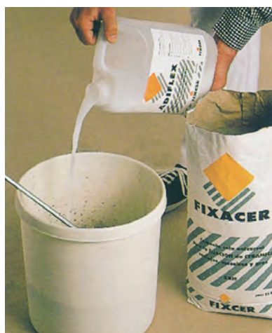
Mixed with FIXACER flexible, very high-performance adhesive is obtained.
