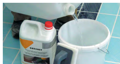
Dilution of GRESNET with water to 1:10.
