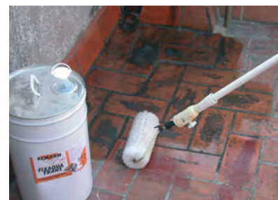
...airless sprayer, brush or roller, preferably with 2 coats
