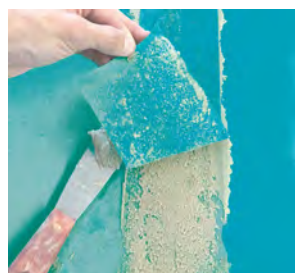
Apply EPOXICOL between the sheets of LAMINAS to attach the BANDA-SOLAPES waterproofing strips.
