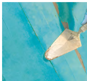
Press firmly on the BANDA-SOLAPES with a smooth-edged trowel.
