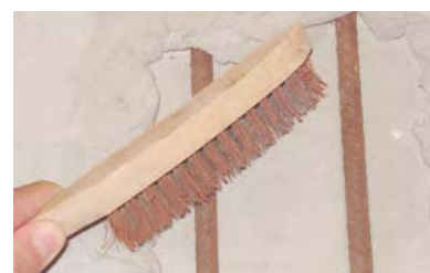
Merely remove any rust encrustations before applying ANTI-OXID LIQUID
