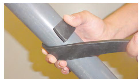
Put FUGA-STOP MINI around the PVC tube ...
