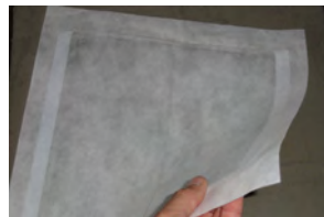
Place the sheet in the center of the sump to be sealed.
