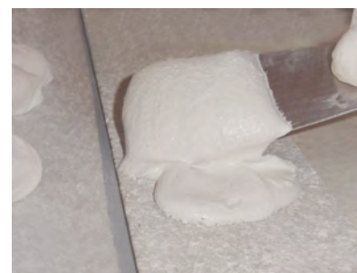
Mix p.ex. the EPOXICOL and apply a layer of 1 - 2 mm up to the masking tape.
