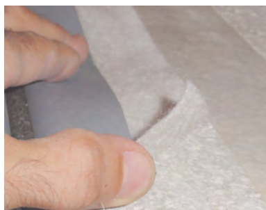
The masking tape should be around 2 cm from the strip.
