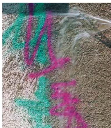
After 5-10 minutes, clean thoroughly with high-pressure water.
