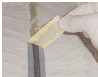
Remove the self-adhesive tape from both sides and also remove the central strip.
