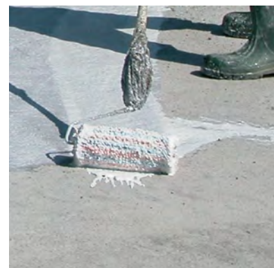
It is applied very easily with a longhaired roller.
