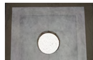
... we will have the surface ready to receive the waterproofing.
