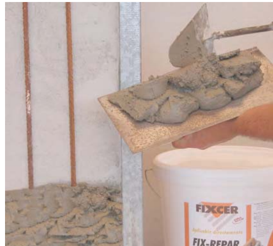
When the ANTI-OXID LIQUID has dried completely, FIX-REPAR R2 or R4 repairing mortar can be applied.
