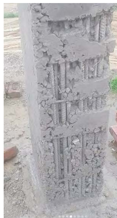
An essential preparatory step for any concrete repair.
