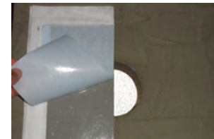
Remove the protective paper from only one of the two parts.
