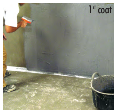
Applying a 1 st coat of HIDROELASTIC.
