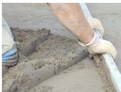
Regularized with a level.
