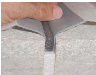
Place the strip along the centre of the joint and make a pleat to be filled with SELLALASTIC FOAM .
