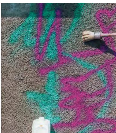
Apply an even layer of un-diluted product with a brush.
