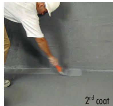
Applying a 2 nd coat of IMPERTOT.
