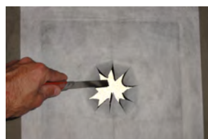
Cut the entire sheet completely discovering the sump.
