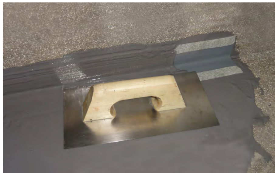
BANDA IMPERMEABLE 120/70 will stick to the surface using cement glue, waterproofing or impermeable paint, as being used in each case.
