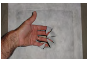
The cuts should start at the perimeter and should reach the center of the drain.
