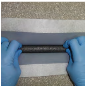
Position the sealing tape in the centre of the joint pushing the tape inside the gap which will then be filled with SELLALASTIC FOAM .
