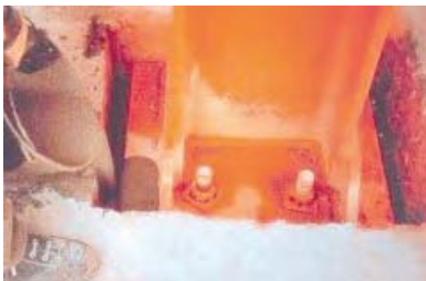
Pour the grout quickly, without stopping.
