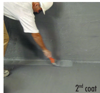
Applying a 2 nd coat of HIDROELASTIC.
