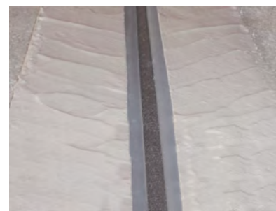
This is the end result: a guaranteed waterproof expansion joint.
