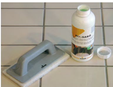
The final cleaning is done the next day with water and FIX-SABO.
