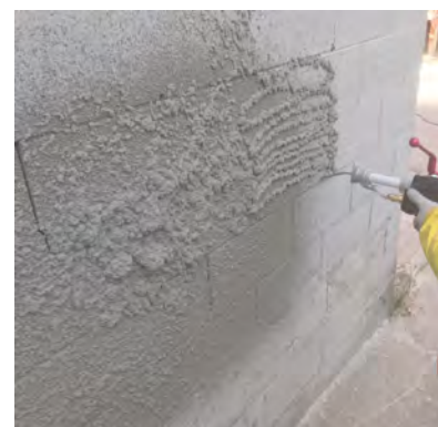
.... start the mortar projection in a way constant and uniform.
