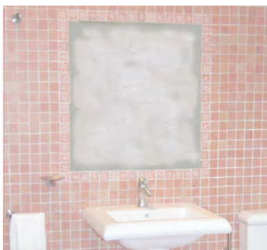
Sealing joints between recessed mirrors and surrounding ceramic.
